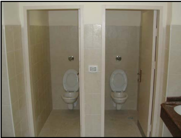
Painting, aluminum windows, lighting fixtures and floor tiles
