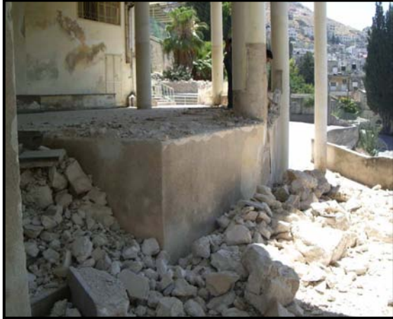
Demolishing the existing parapet
