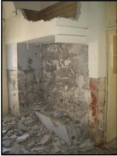
Demolishing Work For the Drinking Water Fountain
