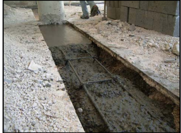
Foundation for block wall
