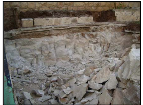
Excavation Works To Reduce Level For Ext. W.C.
