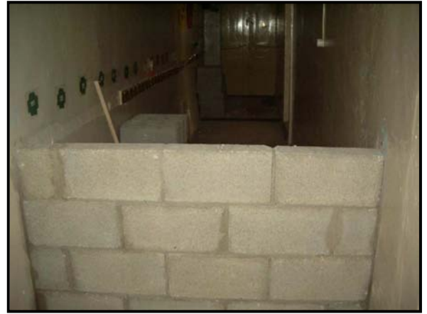
Block Work (store/WC)
