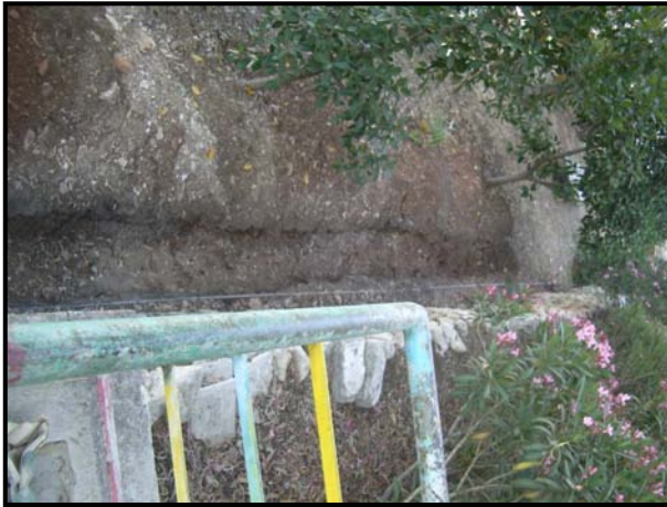
Excavation Work For The External Sewage Line
